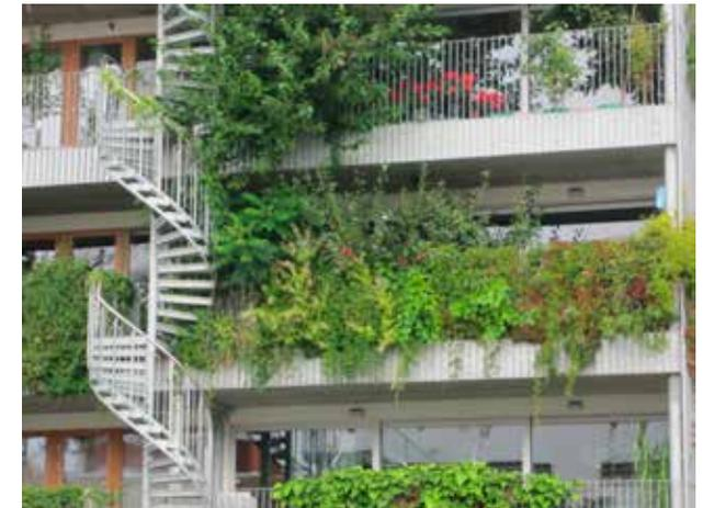
"Urban villas", Malmö. The balconies are reinforced for cultivation beds. There is 30 cm of soil under the floor boards. Any number of boards can be removed in order to access the soil for gardening. (Photo: Varis Bokalders)
